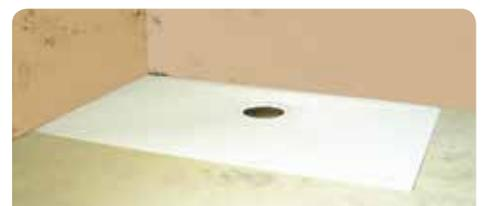
Remove part of existing floor & make the 24mm ShowerDec® absolutely level using plywood.
